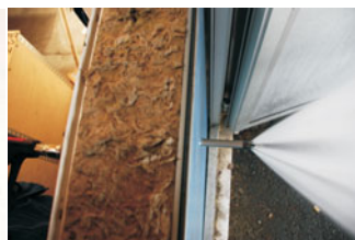
PUNCH THROUGH WALL NOZZLE
